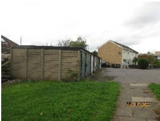
Looking north towards 84 Chilton Drive
