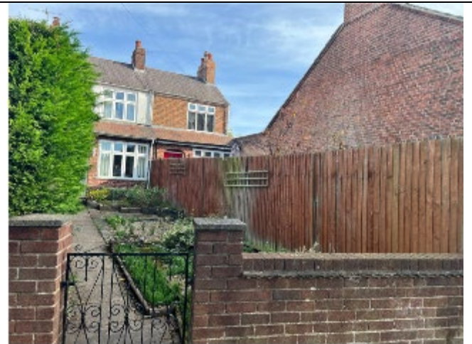
Photograph showing the principle (south west) elevation and the existing extension
