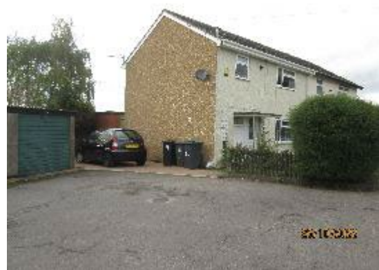
84 Chilton Drive and parking
