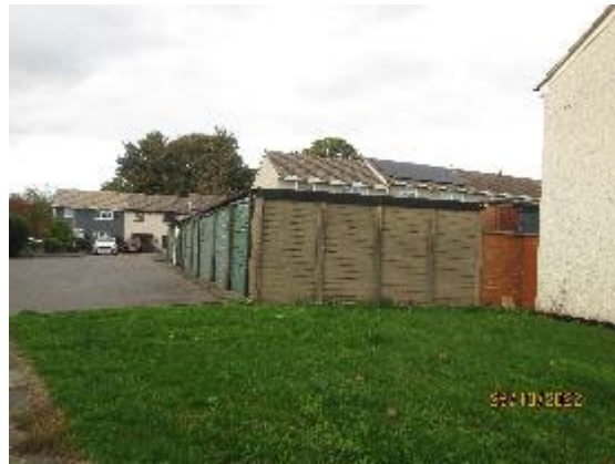
Looking north east towards 61 Chilton Drive
