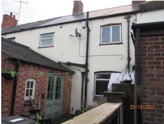
Rear elevation of the adjoining neighbour
